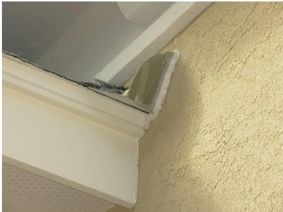
Kick out flashing at roof/wall intersections
