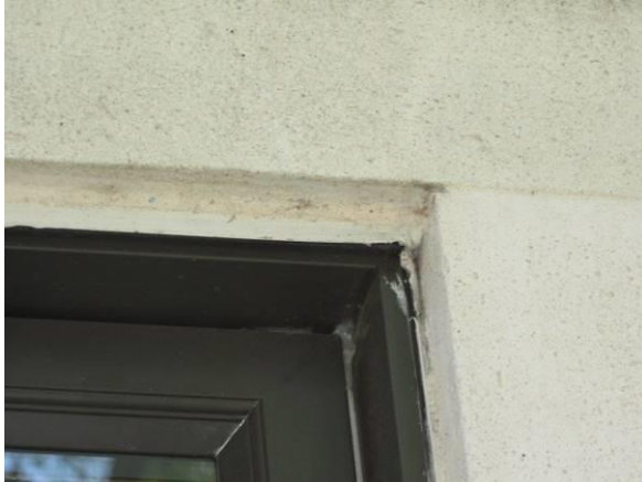
Metal head flashing at top of windows
